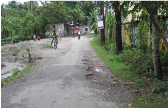
View of road PDP-0072
