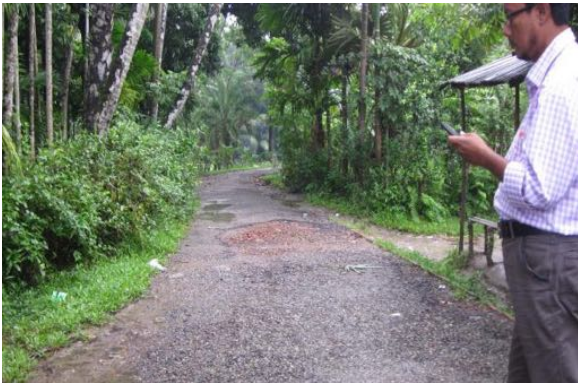
View of road PDP-0026
