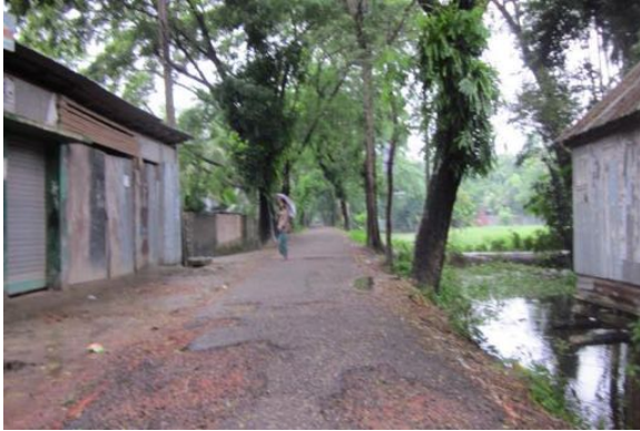
View of road PDP-0034
