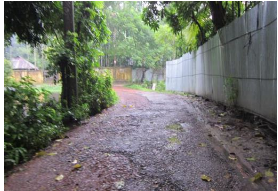
View of road PDP-0014
