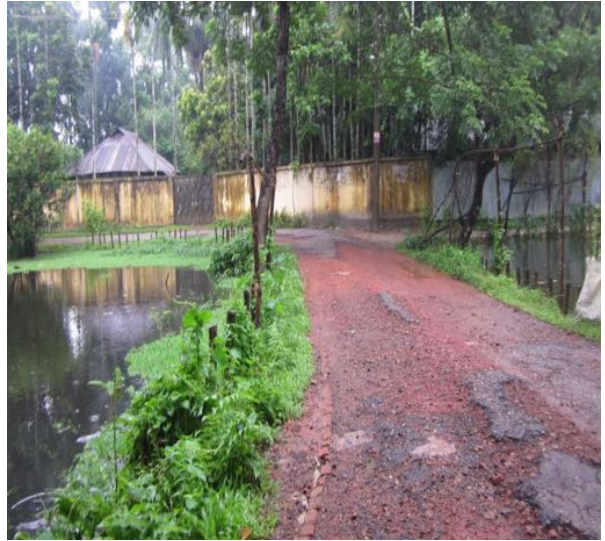
View of road PDP-0040
