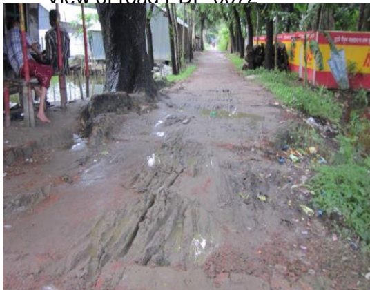
View of road PDP-0076
