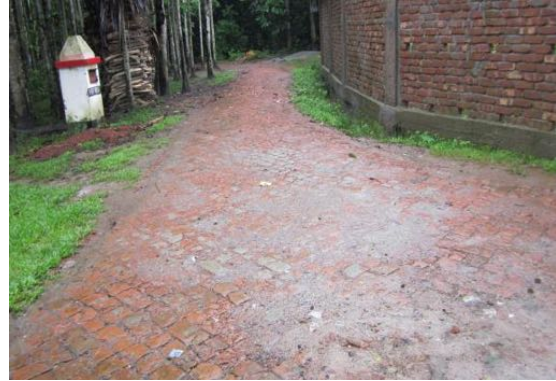
View of road PDP-0042
