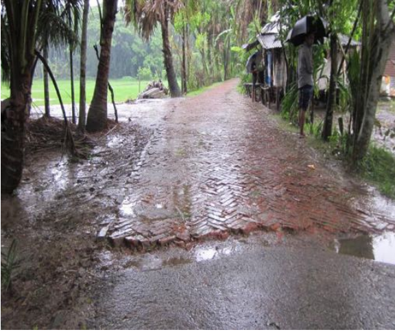
View of road PDP-0003
