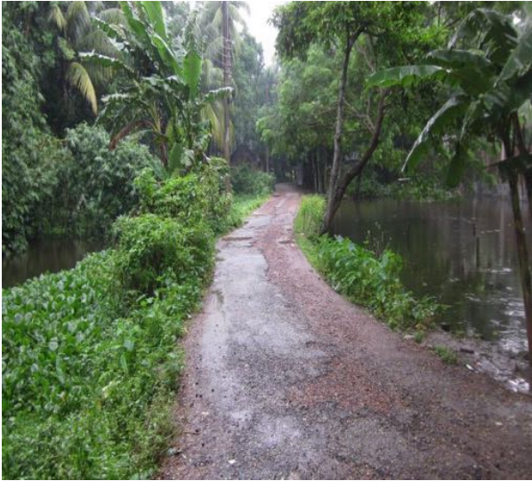
View of road PDP-0034
