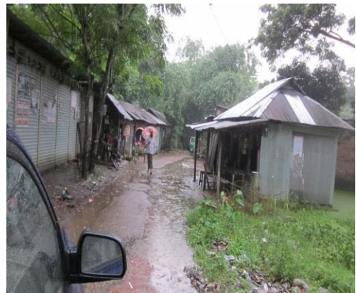
View of road PDP-0025
