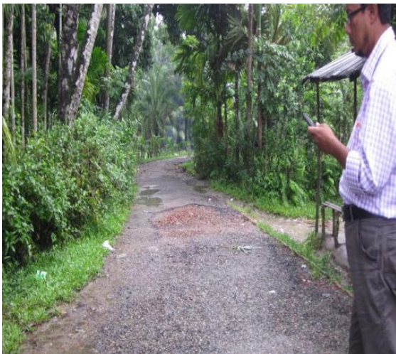
View of road PDP-0018
