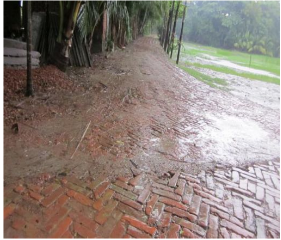
View of road PDP-0004
